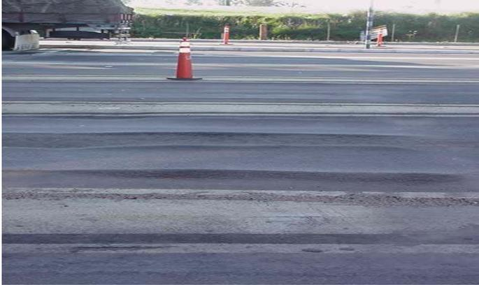
Figure 1. Rutting occurrence in a flexible pavement loaded by heavy traffic
